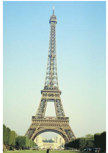
Engineer Gustav Eiffel copied the curved structure of the thighbone to give strength to his famous tower in Paris, France
